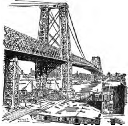
NEW STEEL TOWER BRIDGE ACROSS THE EAST RIVER, NEW YORK.
